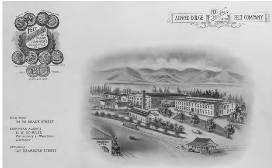
Alfred Dolge Felt Company Publication, showing the factory at the former San Gabriel Winery Property, fronted by the Southern Pacific Railroad and the Pacific Electric Railroad, 1909. Huntington Library.
