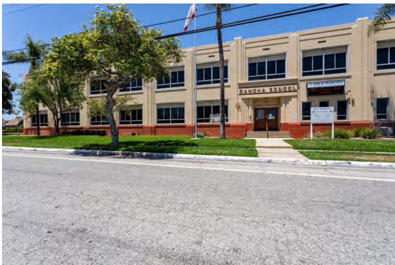
Ramona Elementary School, 509 W. Norwood Place
