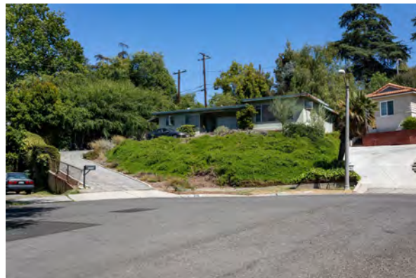
2316 S. Electric Avenue (1952)
