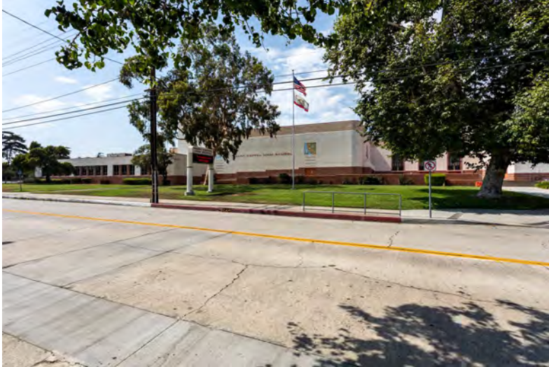
Mark Keppel High School, 501 E. Hellman Avenue (1940)
