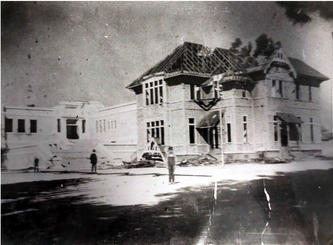
Garfield School, existing school building (foreground) and new building under construction (background left), circa 1909. Alhambra Historical Society Museum.
