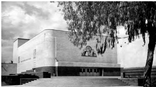
Mark Keppel High School, circa 1940. Alhambra Preservation Group.
