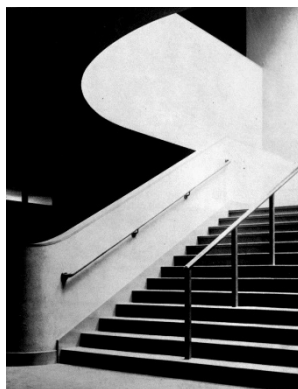
Interior, Mark Keppel High School, circa 1940. Alhambra Preservation Group.
