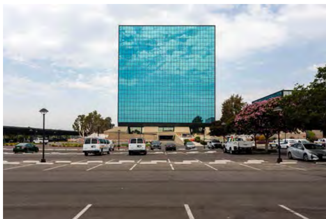
Sears, Roebuck & Co. Pacific Coast Territory Administrative Offices Tower, 900 S. Fremont Avenue (A.C. Martin & Associates; 1971)
