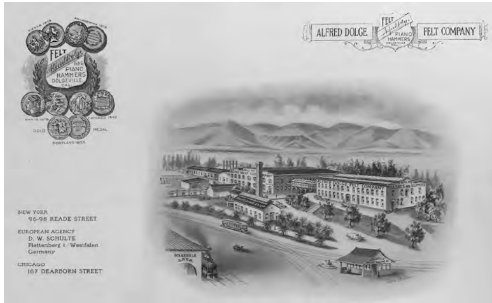
Alfred Dolge Felt Company Publication, showing the factory at the former San Gabriel Winery Property, fronted by the Southern Pacific Railroad and the Pacific Electric Railroad, 1909. Huntington Library.
