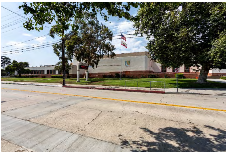
Mark Keppel High School, 501 E. Hellman Avenue (1940)
