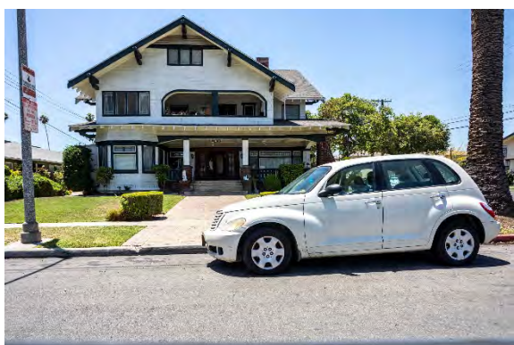
Fred W. Marshall Residence, 1601 S. 4 th Street (1907)
