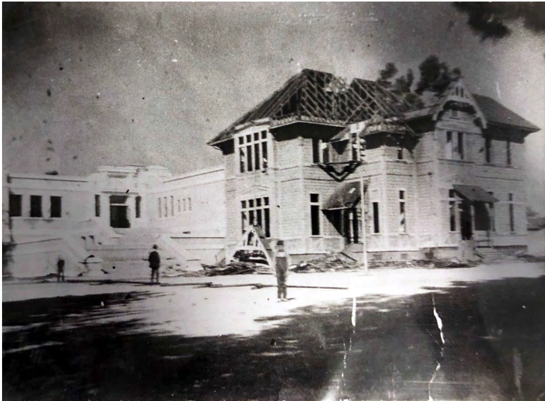
Garfield School, existing school building (foreground) and new building under construction (background left), circa 1909. Alhambra Historical Society Museum.
