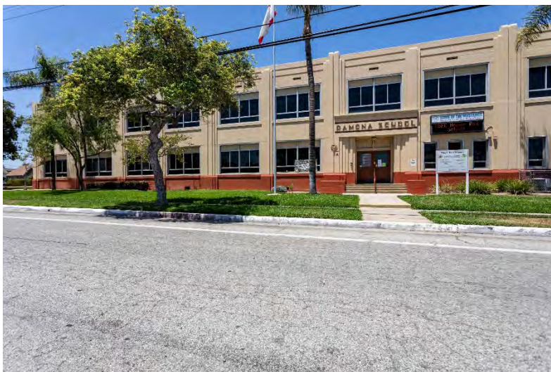
Ramona Elementary School, 509 W. Norwood Place (1936)
