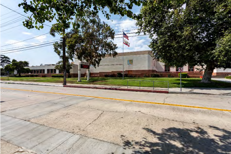
Mark Keppel High School, 501 E. Hellman Avenue (1940)
