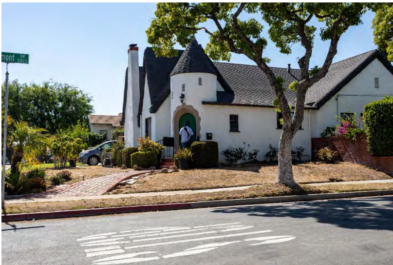
3201 W. Commonwealth Ave (1930)
