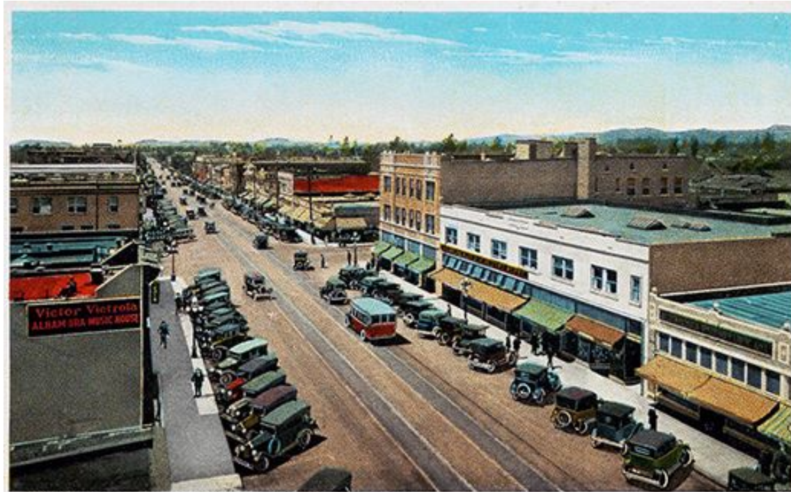
LOOKING WEST ON MAIN STREET, ALHAMBRA, CALIFORNIA.
