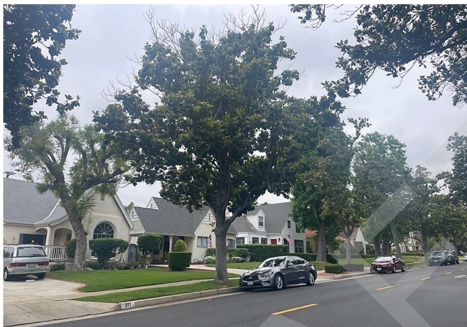
Figure 9. Context view of the Lindaraxa Park-Orange Blossom Manor Potential Residential Historic District. ARG, 2023.
